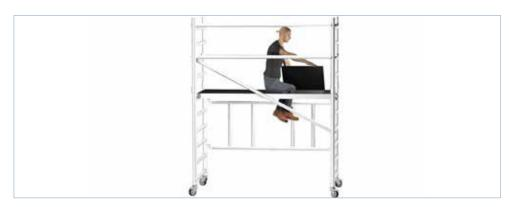
1.14 Fit the toe boards into place, then the erection of the LEWIS 1.6m platform height Miniscaff is complete.
